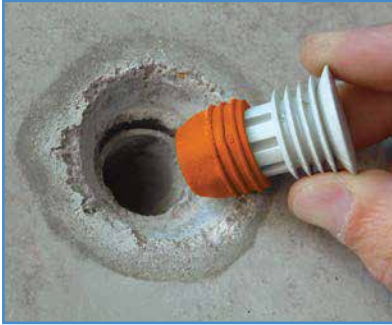
1. Insert the CJ Form-Tie Plug into the hole.
