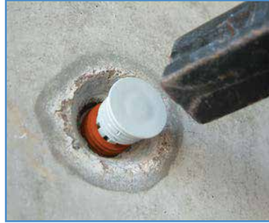
2. Hammer the CJ Form-Tie Plug into the hole.
