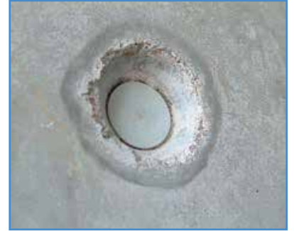
3. The CJ Form-Tie Plug completely installed.
